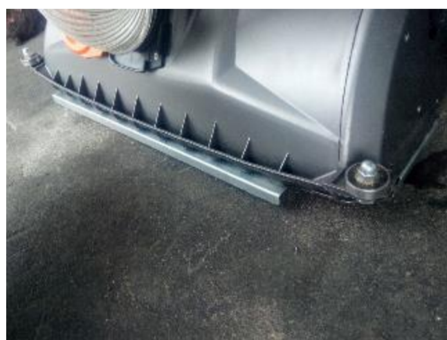
Fig.30-2 The baffle is inserted into place
